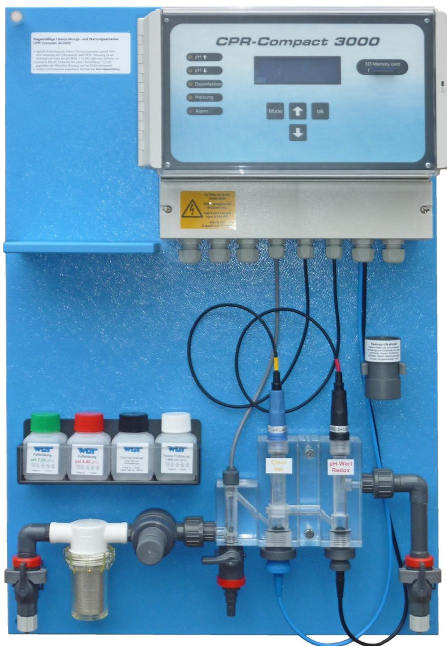
**Auto-Control System for free Chlorine, pH-value and ORP/Redox-tension, temperature**
